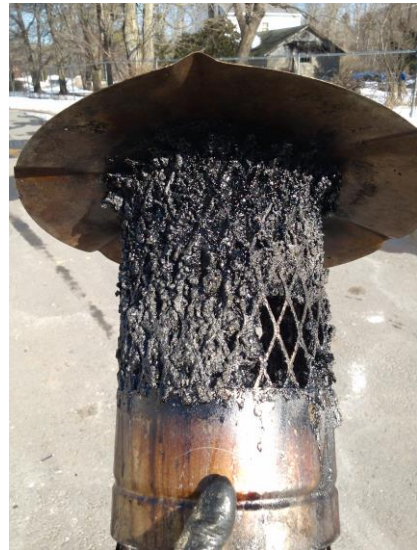
Figure 18 - Tared up chimney bird guard
