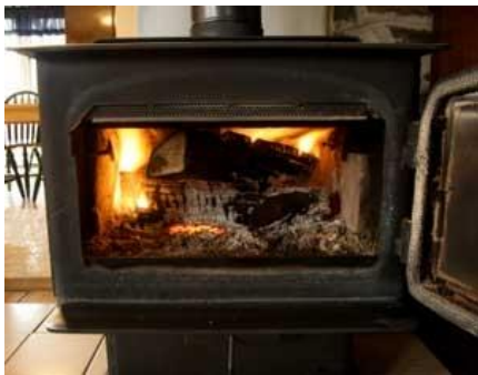
Figure 5 - Example of a wood / log burning stove with no ash-pan
