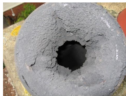
Figure 14 - Chimney sweeping annulus
