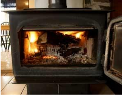
Example of a wood / log burning stove with no ash-pan
