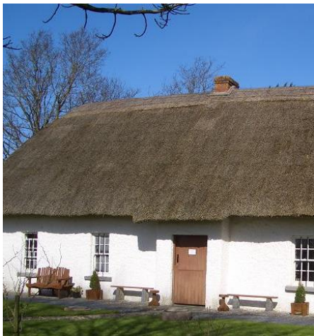
Figure 11 - Thatched property with very small pot top to thatch clearance
