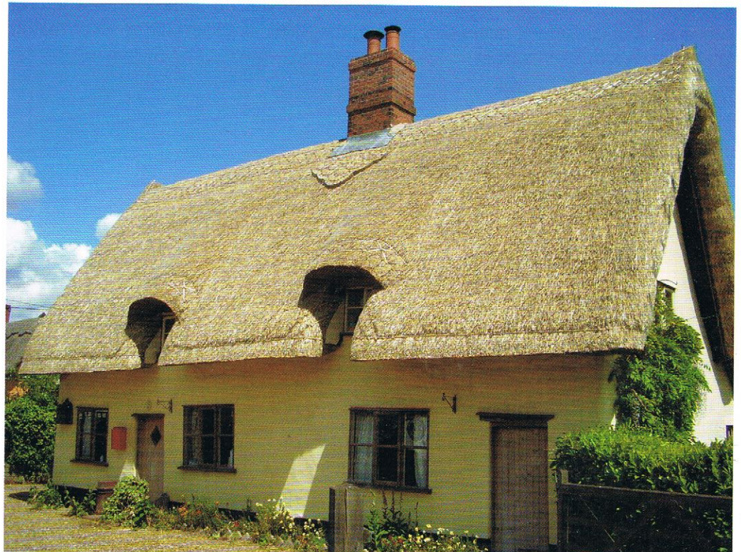
Figure 9. Typical authentic Norfolk long-straw thatch (in Pulham St Mary) with a flush ridge finish, as seen commonly before the mid-20th century.
