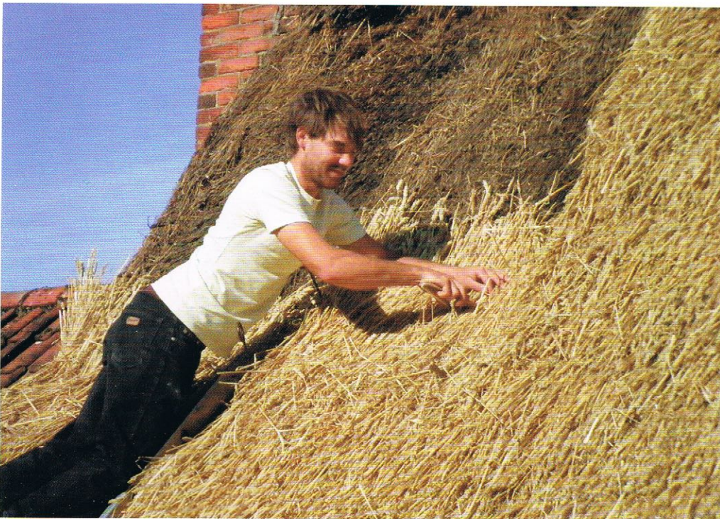
Figure 7. The author's former apprentice, Bodkin Willows, fixing new long straw thatch to an existing coat of thatch using hazel brotches (staples).
